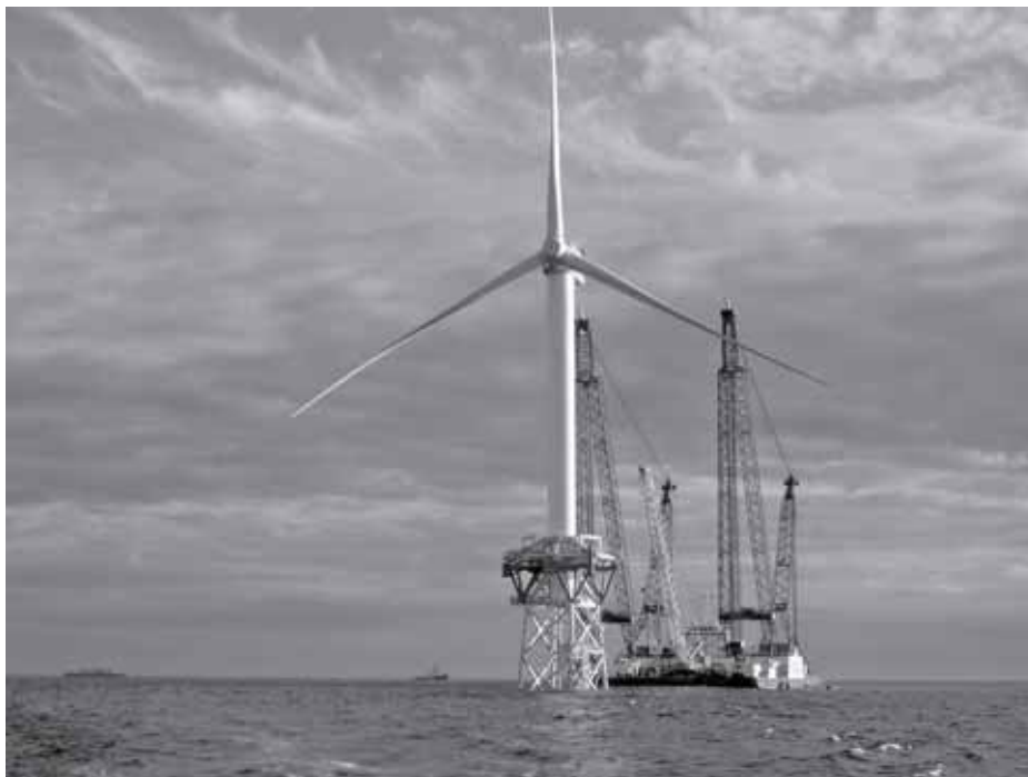
Figure 5 REpower 5M installed on a jacket foundation in the Scottish North Sea in August 2006. Source: REpower Systems Inc.
