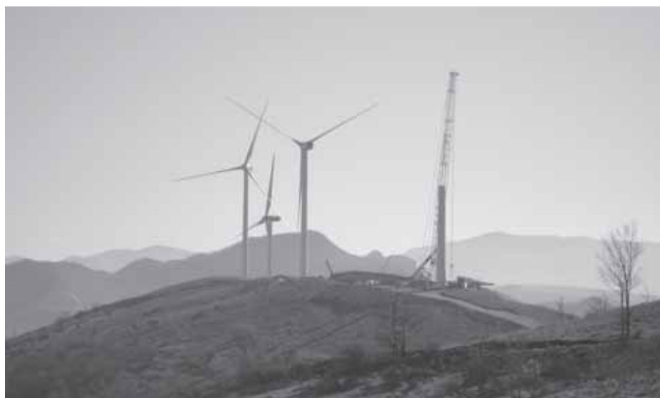
Figure 7 Vestas V90 3-MW turbines at Ricigliano in the Campania region, a 36-MW wind farm developed by FRI-EL
