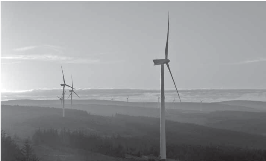
Figure 2 Kilgarvan, County Kerry 3-MW wind turbines. Courtesy of T. J. Hunter.
