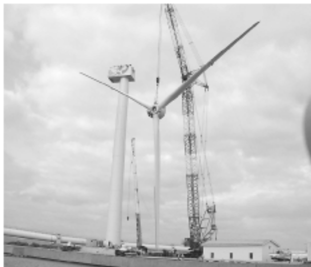
Figure 12.2 Mitsubishi's MWT-S2000 wind turbine under construction at Gushikawa in Okinawa
