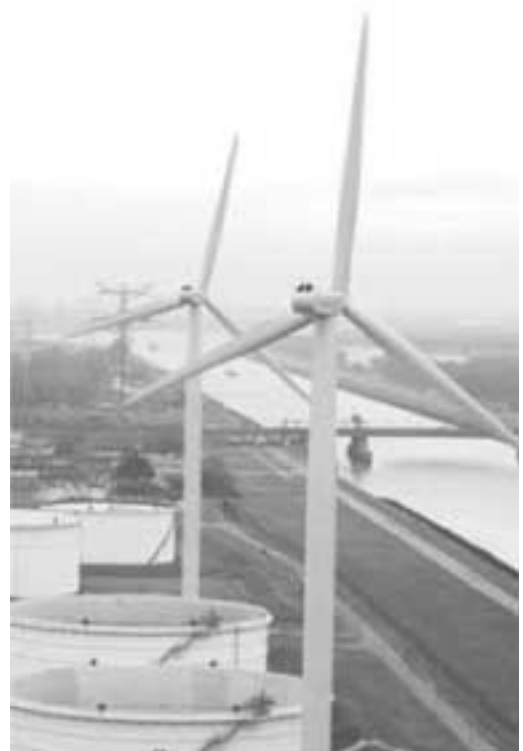
Figure 14.3 2.5-MW wind turbines at Nerefco refinery
