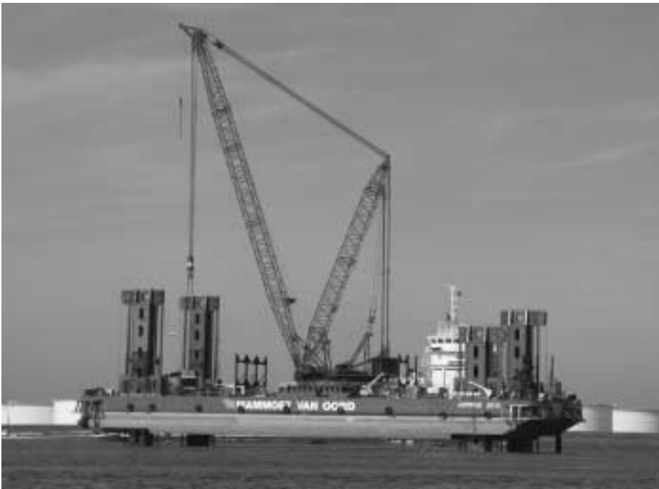
Figure 14.5 Jumping Jack offshore installation barge
