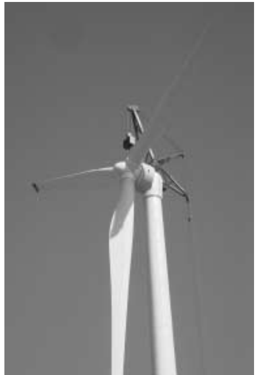
Figure 14.4 Erection of Lagerwey 1.5 to 2 MW prototype
