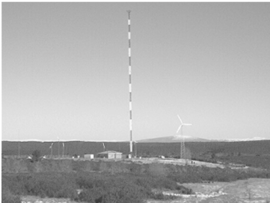
Figure 17.8 CEDER-CIEMAT test plant
