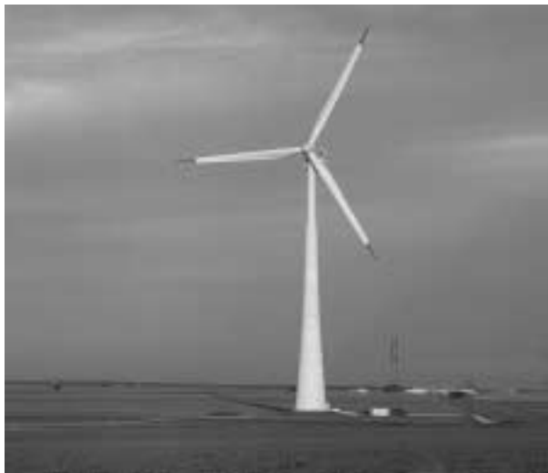
Figure 17.7 GE Wind Energy 3.6-MW prototype (Barrax-Albacete)
