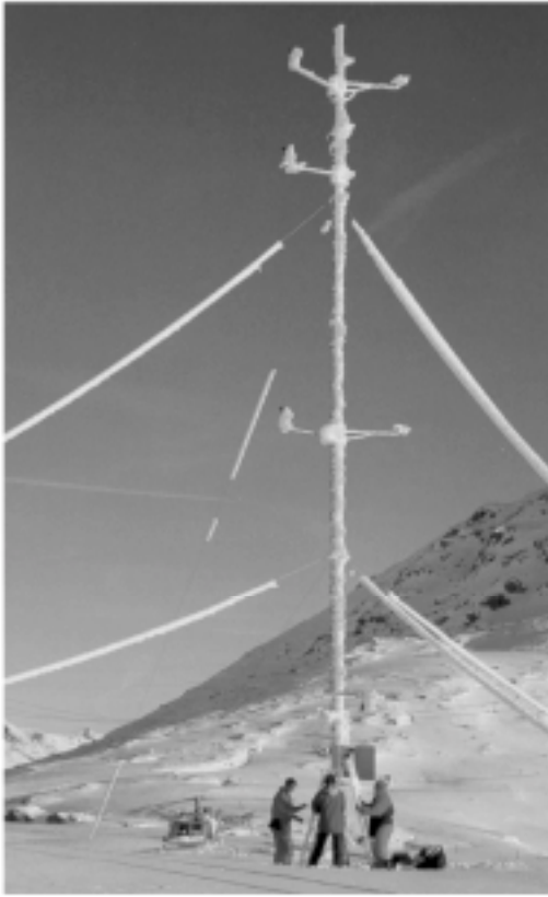
Figure 19.5 and Figure 19.6 At low temperatures, ice and snow accumulates on the mast and guy wires leading to greater loads and a larger area of attack for gusts (photos taken from a Meteotest measurement campaign on the Gotthard Pass at 2,100 m above sea level, Switzerland, courtesy NEK Umwelttechnik AG)
