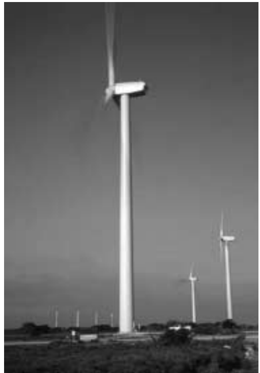
Figure 21.1 GE Wind Energy 1.5-MW turbines in 150-MW Trent Mesa wind-power plant located near Sweetwater, Texas
