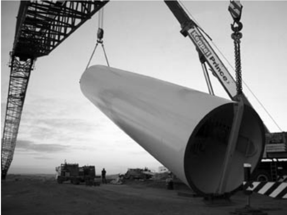
Figure 4.1 Tower construction at Challicum Hills wind farm Image courtesy Keppel Prince
