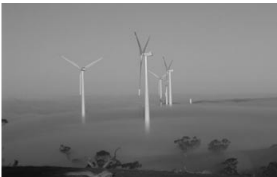
Figure 4.2 Mist below Chalicum Hills wind farm during construction Image courtesy Keppel Prince
