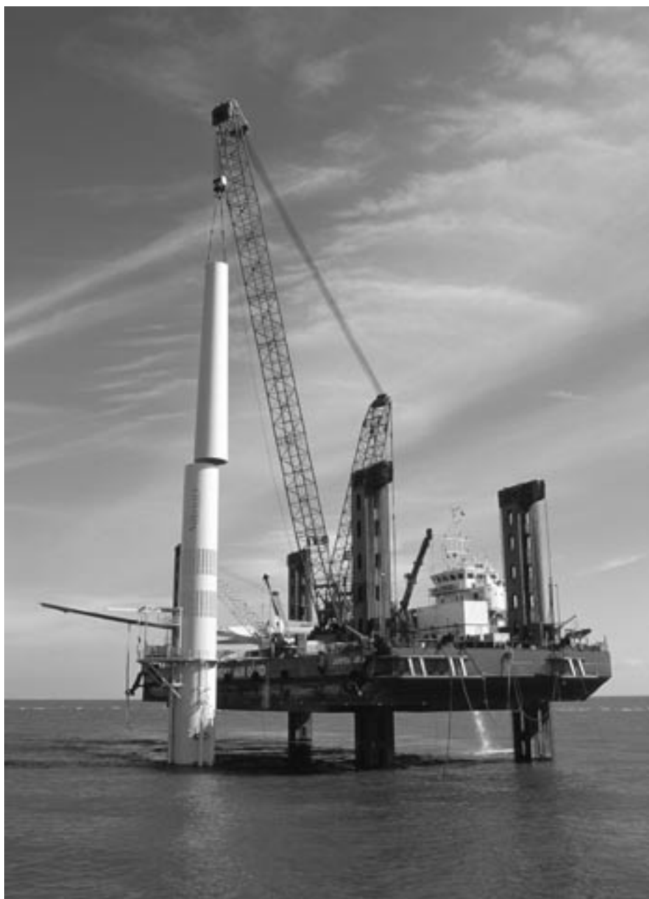
Figure 10.1 Tower construction offshore in Ireland (Courtesy of Airtricity)
