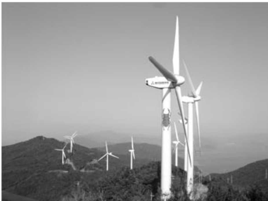
Figure 12.4 A large wind farm in Japan
