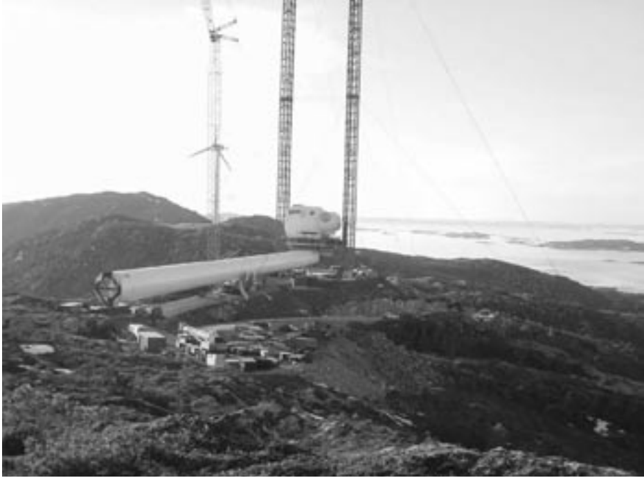
Figure 15.1 Erection phase for the direct-driven ScanWind 3000 DL turbine at Hundhammerfjellet
