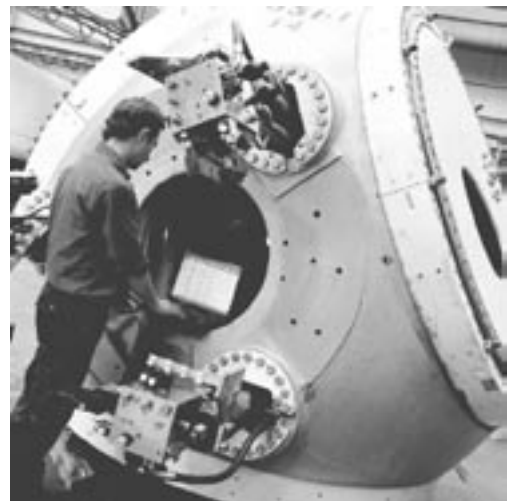
Figure 17.9 Manufacturing of a hub by Gamesa
